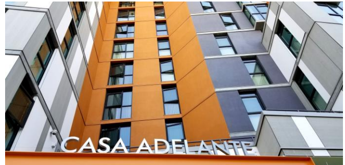
Figure 18 - Entrance to the building
