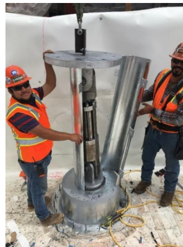
Figure 16 - Lead extrusion dampers being installed in the mat slab
